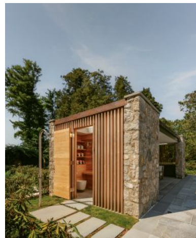
On axis with the rear terrace, a trim pool house includes a cedar-lined changing room in the louvered side façade.
